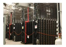
Notrees Wind Farm Project, West Texas: Xtreme Power's (36MW x 15 minutes) battery based energy storage system at Duke Energy's 153MW wind farm.
