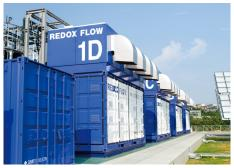
Yokohama Smart City project, Japan: Sumitomo Electric's redox flow battery (1MW x 5 hours) located at Sumitomo Electric Industries (SEI) facility, links the world's largest redox flow battery with Japan's largest concentrated PV array
