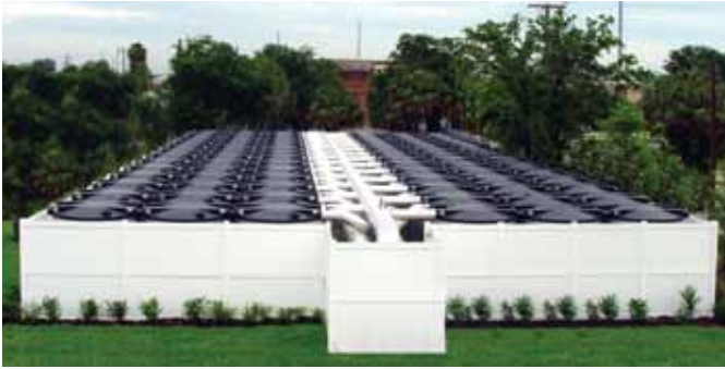
⤴ Figure 5 A system like this, consisting of several storage tanks, can shift more than 2 MW of electrical power consumption to nighttime.
