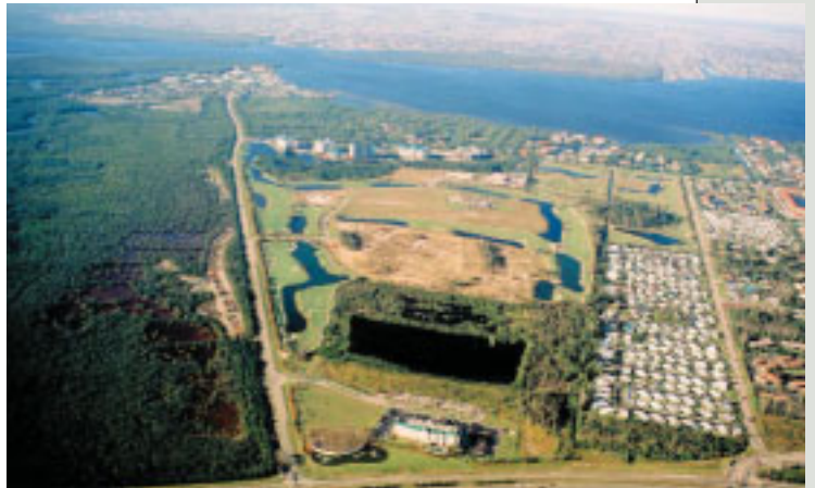
Aerial view of Shell Point Retirement Community.
