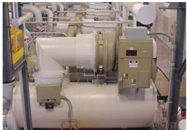
Green Seal-certified low-pressure Trane CenTraVac
